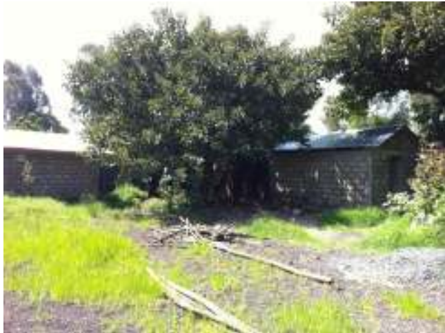
Toilets newly built for girls and boys separately
